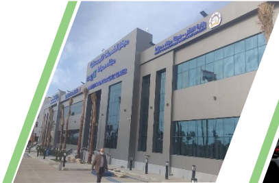
DAMIETTA PORT LOGISTICS CENTER
