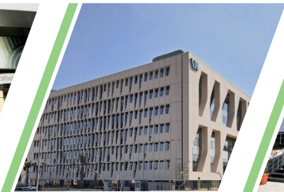
ABC BANK HEADQUARTERS
