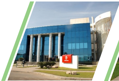
VODAFONE SMART VILLAGE
